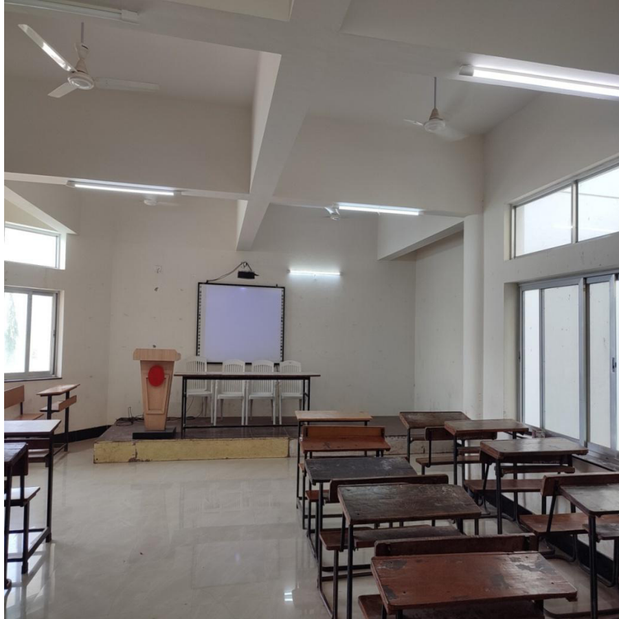
Fig. 4. : Existing Lighting System
