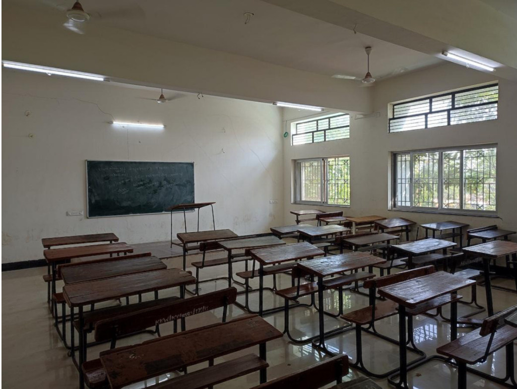
Fig. 3. : Conventional Ballast FTL
